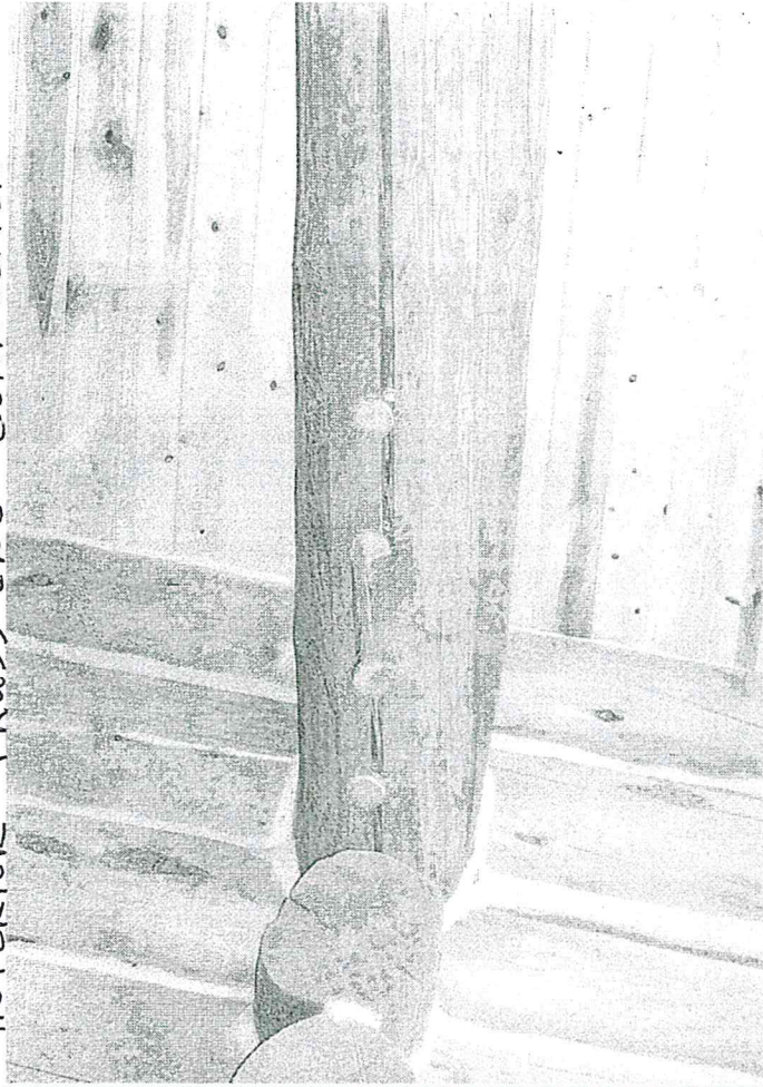
UNDERSIZED AND TWISTED PURLIN: UNSUITED FOR ANY STRUCTURAL GRADE
