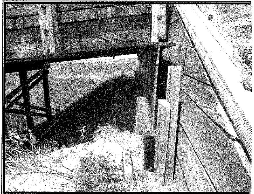
Rotated East Abutment Cap
